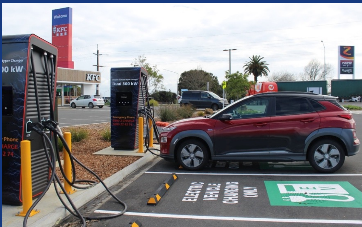
Image courtesy of ChargeNet NZ. EV charging site Ross Holdings, Bombay New Zealand.
