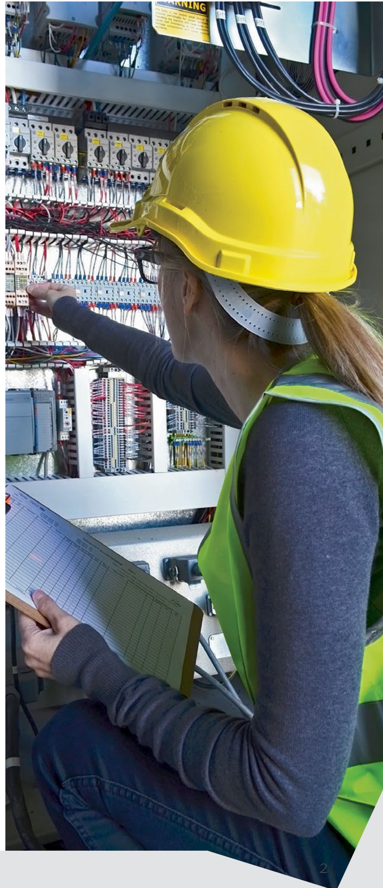
Voltage optimisation (credit: iStock)
