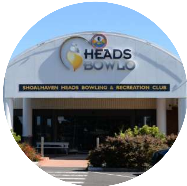
Shoalhaven Bowling Club, which has installed 99 kW of community-owned solar through support from the Fund for Renew Shoalhaven (Photo: OEH)
