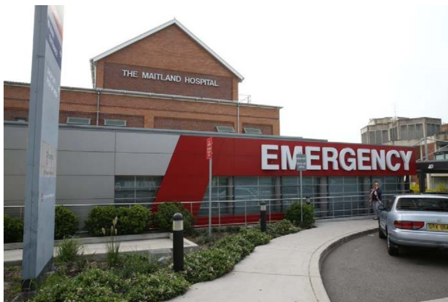
Maitland Hospital in Hunter New England Local Health District (Photo: OEH)
