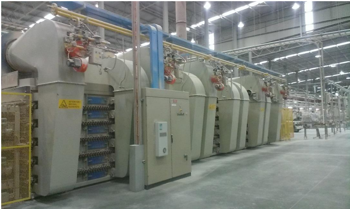
The main kiln where tiles are fired (Photo: Energy Saver, OEH)
