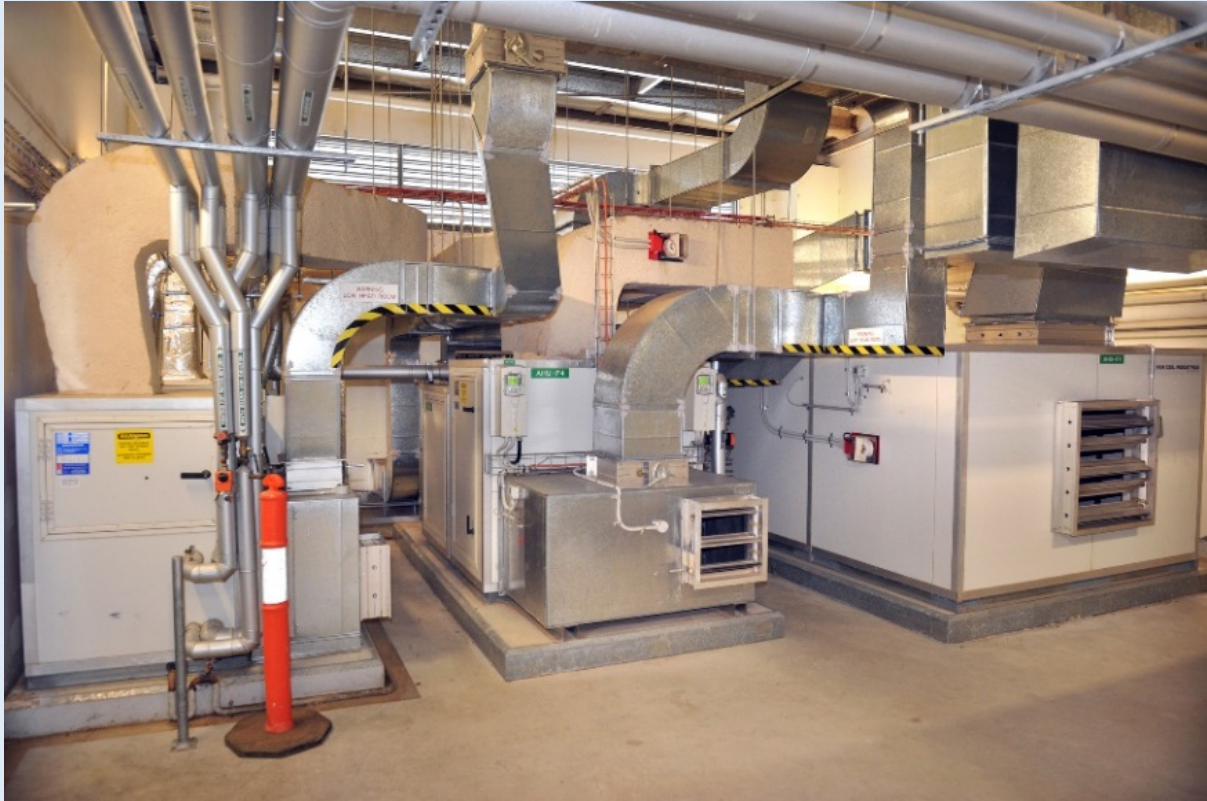
Heating, ventilation and air-conditioning equipment at Queanbeyan Hospital (Energy Saver Program, OEH)
