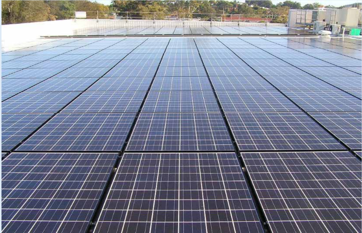
Solar photovoltaic panels (Coffs Harbour City Council)
