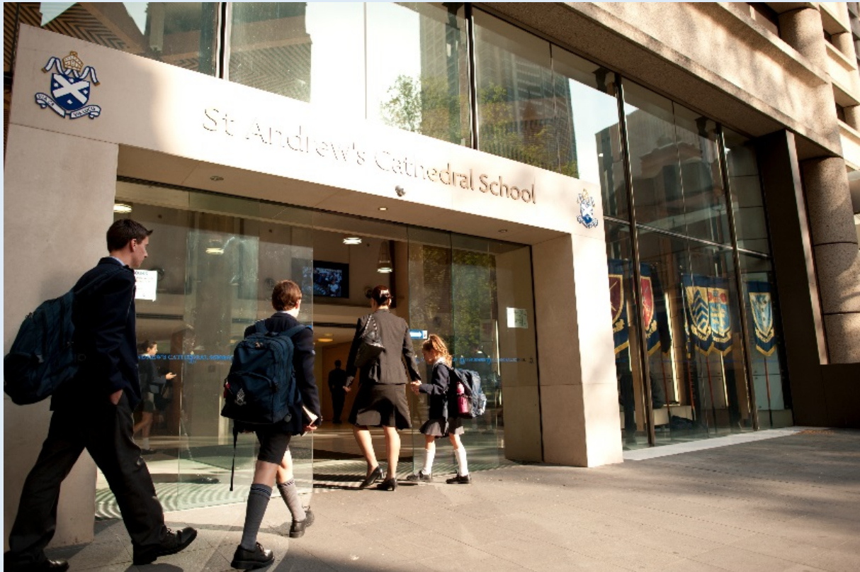
Front of St Andrews Cathedral School (Energy Saver Program, OEH)
