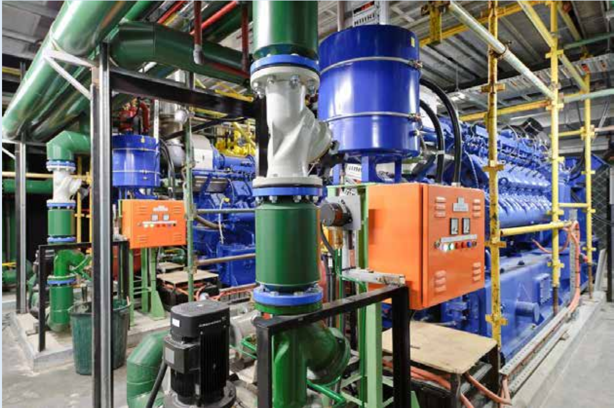
Cogeneration equipment (GPT Group)
