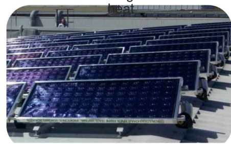
Flat plate: a plate of passaged tubing containing heat transfer liquid
