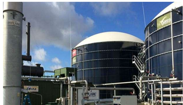
Richgro bioenergy plant – Jandakot, WA
