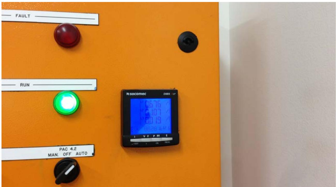
**Figure 3:** Panel meter installed in mechanical switch board
