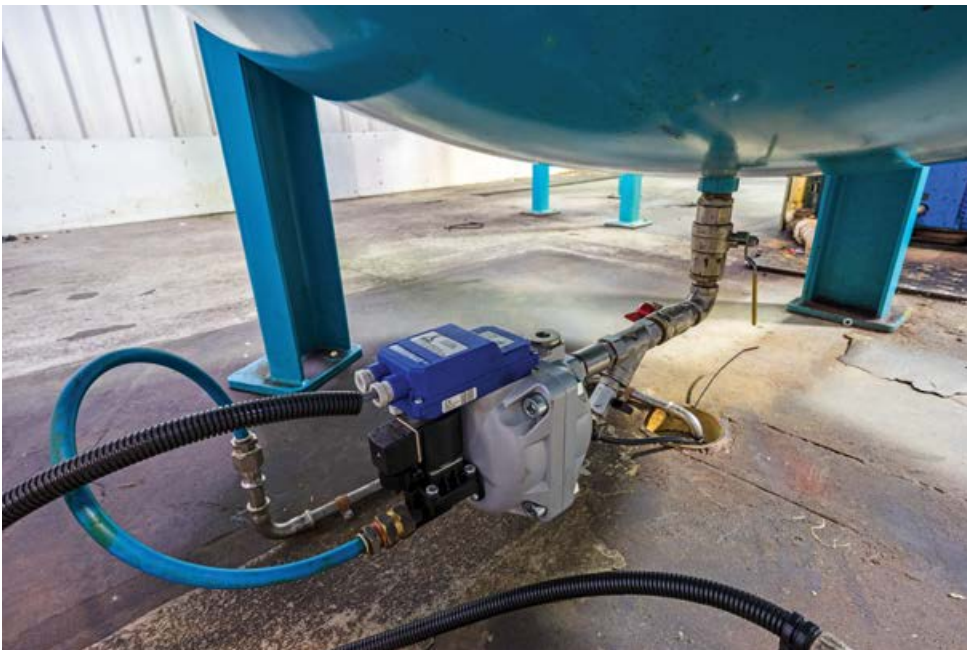
Automatic drain on a receiver tank
