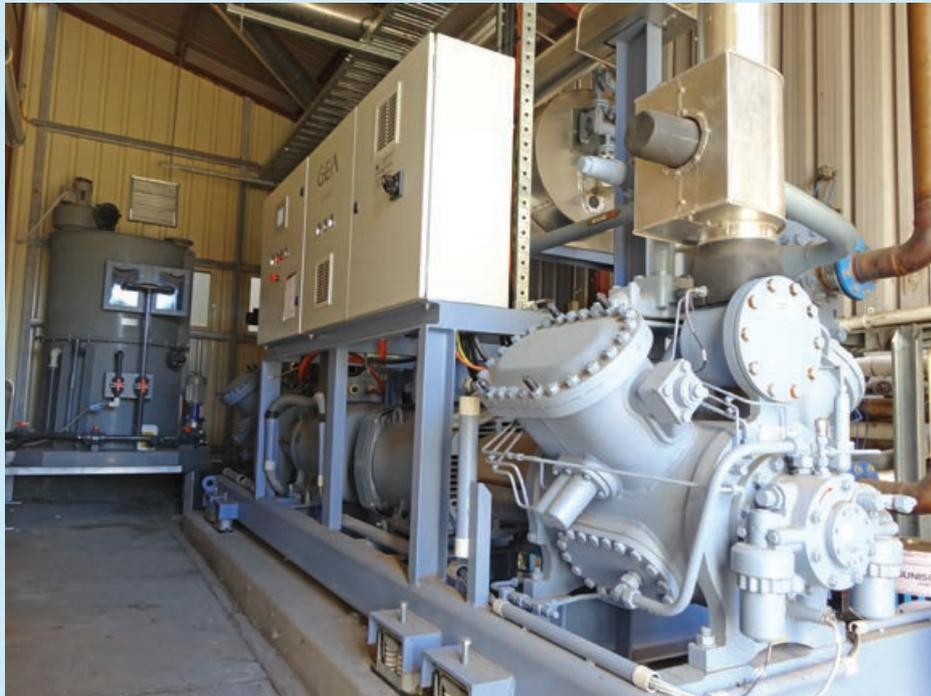
Figure 33: Water-cooled ammonia chiller at Riverina Fresh, Wagga Wagga
