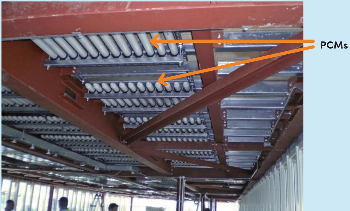
Figure 16: PCMs installed in the ceiling space
