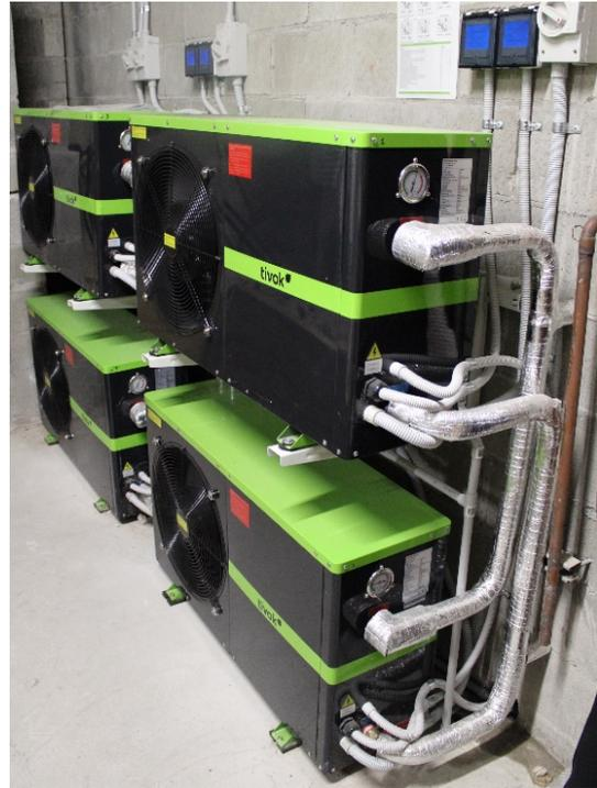
The picture shows heat pumps extracting heat from the air to warm water.
