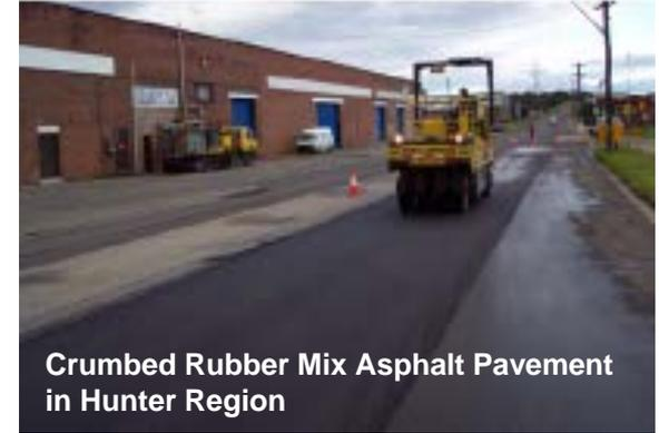
Crumbed Rubber Mix Asphalt Pavement in Hunter Region
