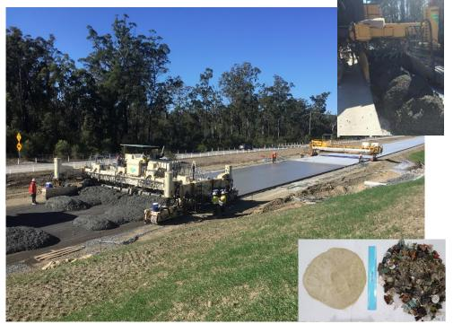
Pacific Highway Woolgoolga to Ballina (W2B) Project (Sub base course & shoulder base concrete with 15% crushed glass)
