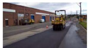
Crumbed Rubber Mix Asphalt Pavement in Hunter Region
