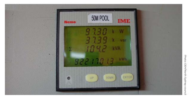
Figure 10: An electrical meter
