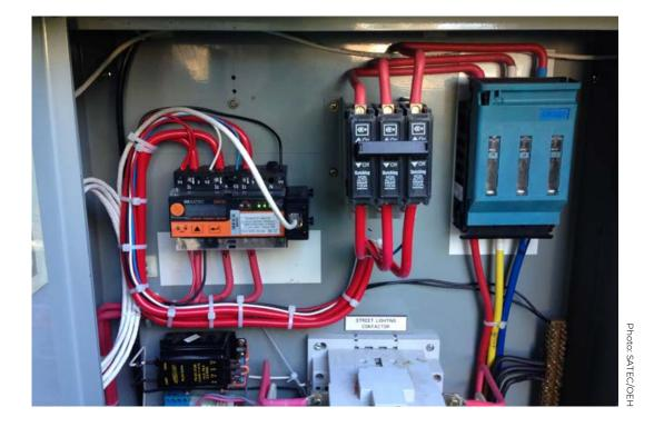
Meters have a constant known as the K factor, which represents the ratio of the energy registered by the meter and the actual human readable output. For solid-state meters this is generally the number of pulses per kilowatt hour.
