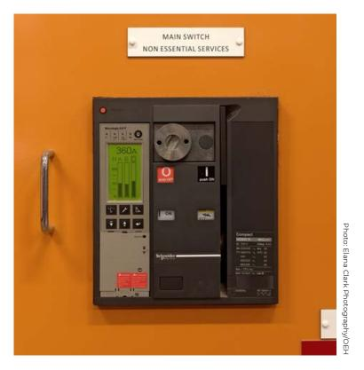
Figure 6: Electronic circuit breaker capable of monitoring electric current.
