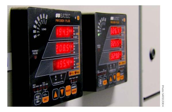
• **direct-connected (whole current) meters** – are directly connected to electrical circuits, with a rated capacity up to 100 amps, which is passed through the meter without a CT.
