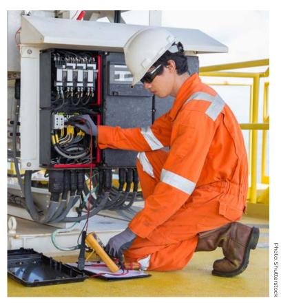
Figure 13: Verifying voltage readings
