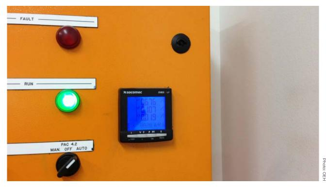
Figure 3: Panel meter installed in mechanical switch board
