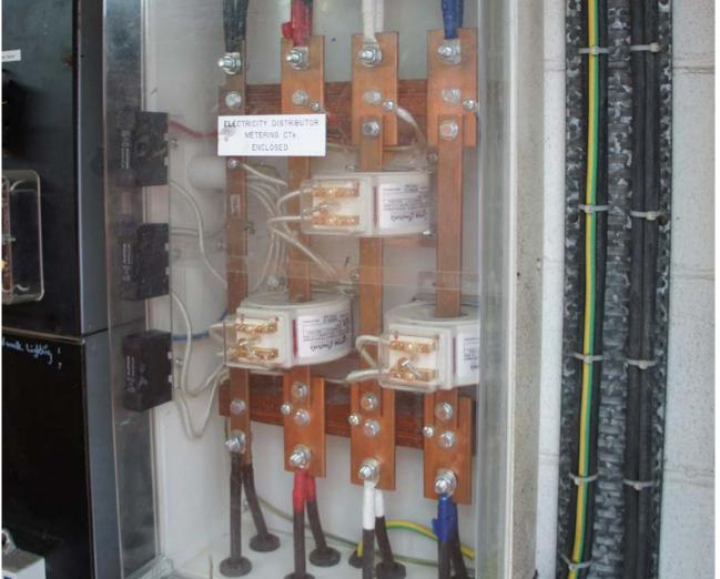
Figure 12: Solid Core CTs around bus bar
