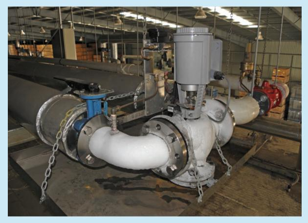
Figure 39: After: a motorised valve installed at the end of the circuit
