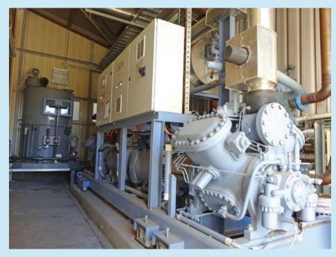
Figure 33: Water-cooled ammonia chiller at Riverina Fresh, Wagga Wagga
