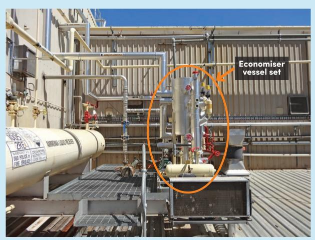
Figure 24: Rivalea's economiser vessel set for condensate sub-cooling
