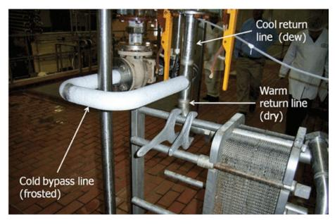
Figure 35: Example of three-way valve control mixing warm and cold fluid streams
