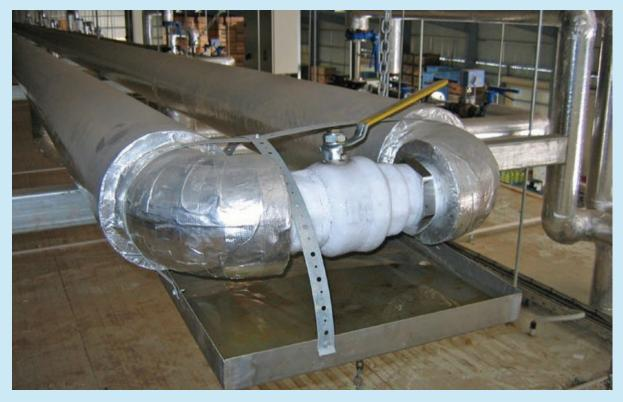
Figure 38: Before: a fully opened ball valve at the end of the circuit to bypass unused flow
