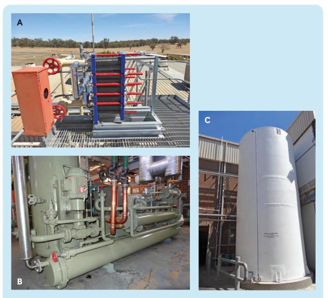
Figure 13: Rivalea Australia's heat recovery system: A. de-superheating heat exchanger, B. heat recovery oil cooler, and C. hot water storage tank Photos: Rivalea Australia/OEH
