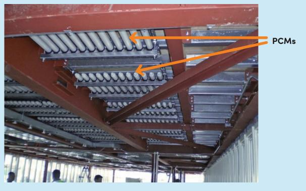
Figure 16: PCMs installed in the ceiling space Photos: OEH
