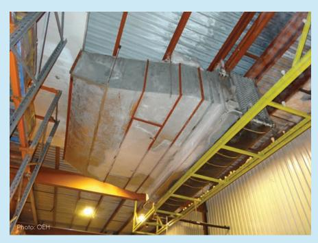
Figure 19: Ammonia evaporators in the Montague Cold Storage cool room
