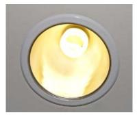
Figure 19: Compact fluorescent replacement lamp in recessed downlight
