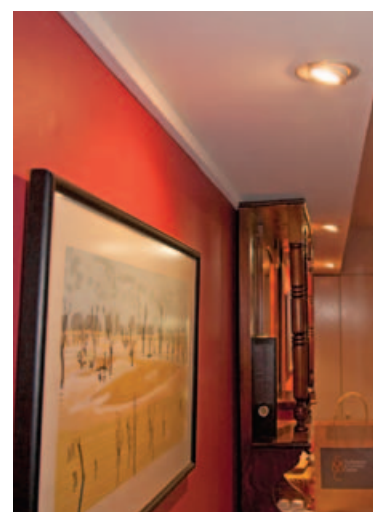
Figure 41: Halogen used to highlight pictures – good practice
