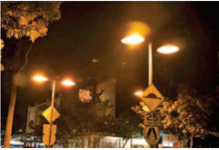
Figure 63: Typical sodium vapour street lights
