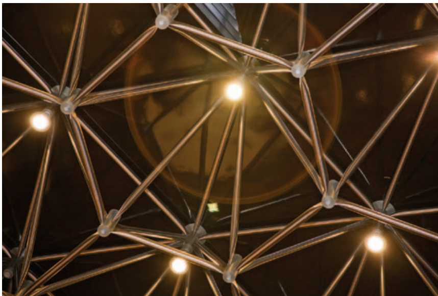
Figure 11: 18 W LED parabolic aluminised reflector (PAR) lamps
