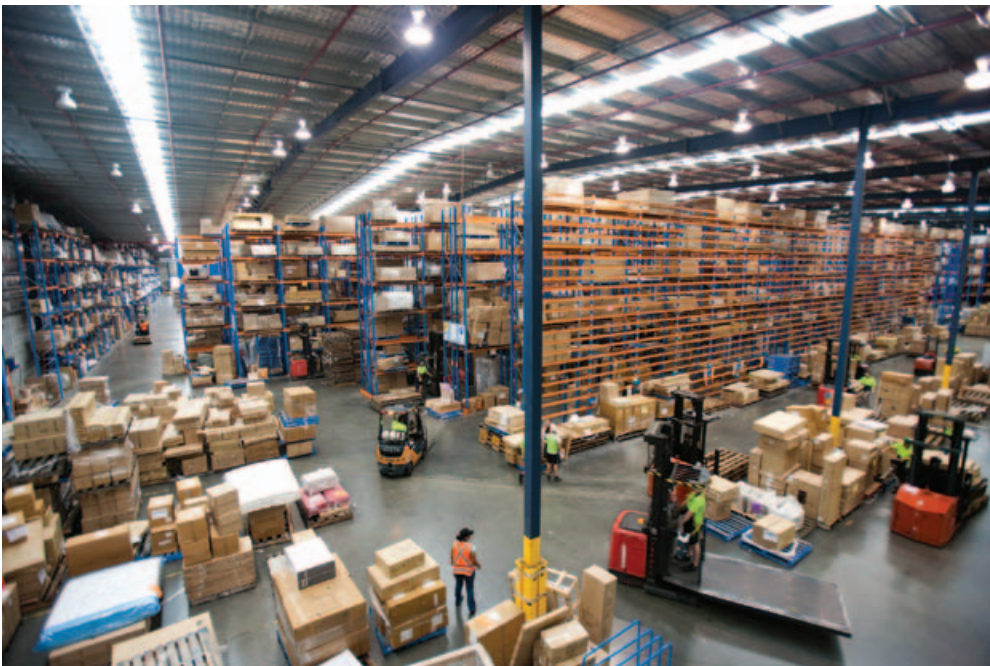
Figure 8: Typical warehouse using high bay lighting technology
