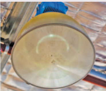
Figure 54: A deteriorating lamp consumes energy while producing minimal light
