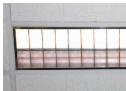
Figure 13: An example of de-lamping, where one tube is taken out of the circuit
