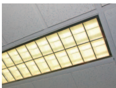
Figure 12: Two of the most common types of recessed troffer fittings. The luminaire above uses a louvre to control the direction of produced light, while the luminaire below uses a diffuser.
